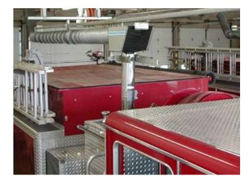
MagnaStack is a fully automatic exhaust extraction system. The extraction unit designed as a hood enclosure automatically connects with the vertical exhaust stack as the vehicle is backed in to the parking bay. Guide arms position the laterally adjustable hood to the stack. The stack is locked to the hood with an electro-magnet.
