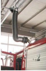
The MagnaTrack HS is designed to serve emergency stations with a high frequency of runs. The track system serves one vehicle at a time. The balancer has a constant liftning power.
