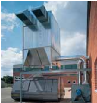
NFS On structure/ Dumping into bin
