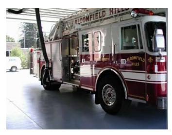
The MagnaTrack S is an economical alternative to MagnaTrack HS designed for a normal frequency of runs and exit speeds. Magnatrack S has an elastic cord inside the exhaust hose (instead of a balancer) and a rubber stop (instead of a hydraulic trolley stop).
